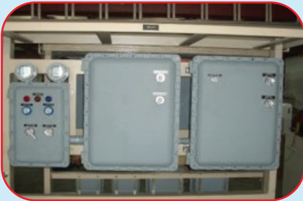
Ex'd IP65 Panel Control
